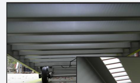
Structure consists of heavy duty formed steel side girders fully welded to high strength steel joists. (Picture shows under side of ramp)
