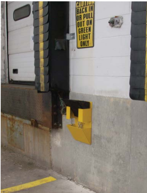
Wheel Chock Cradle, Chock and Chain in Use
