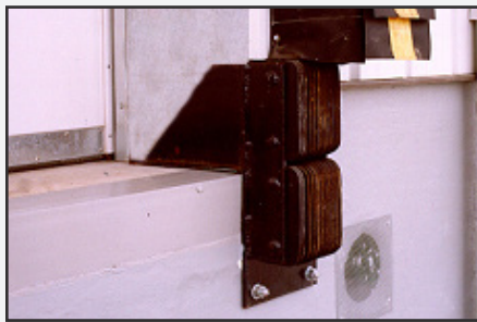
Vertical laminated bumpers with gusseted bracket and load distribution plate.
